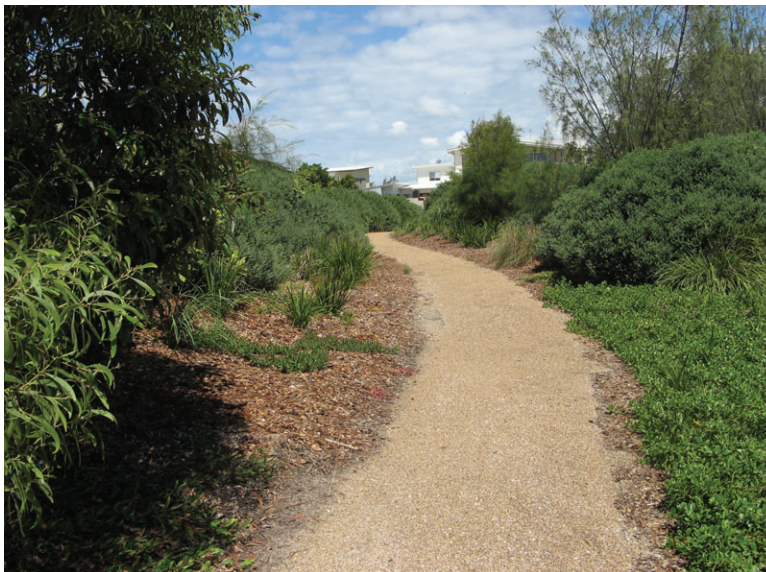
Informal pathway connections from private terraces to the Reserve (located within property boundary). Pathway to be constructed of decomposed granite gravel.
