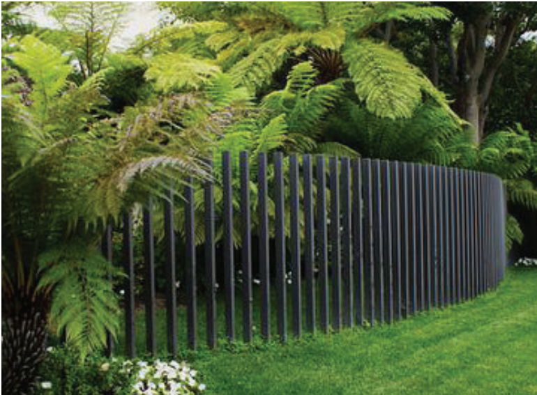
Fencing between terraces and a balustrade will consist of a simple steel blade structure, protective coating system to match architectural steel work.
