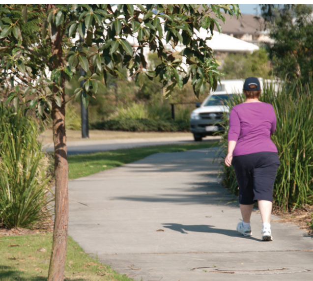
Reinforced concrete pathway with broom finish, 2.0m width. Pathway to be surrounded with robust, low-maintenance native planting and shade trees.
