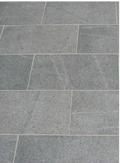
Primary surface treatment to be stone unit paving installed on mortar bedding and reinforced concrete base slab. Contrasting stone colour and texture will be used selectively throughout.
