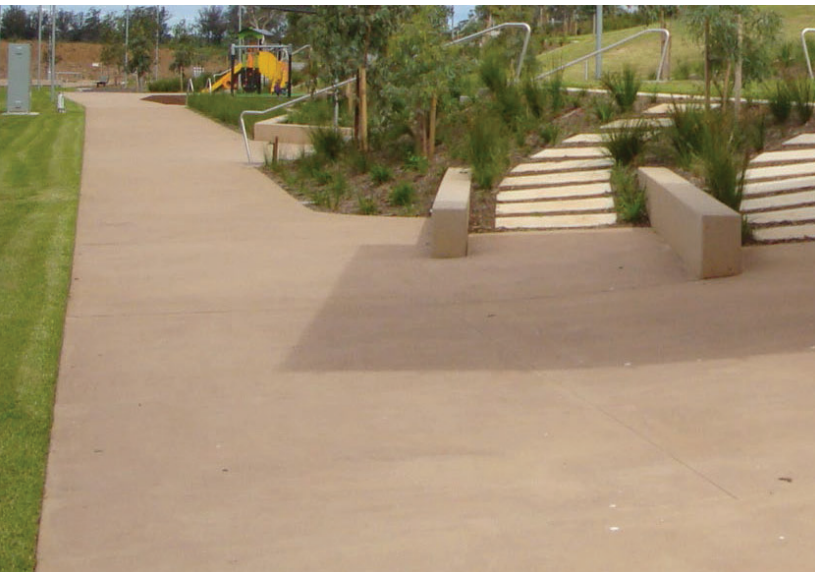
Secondary surface treatment to be reinforced, full depth coloured concrete pathways with lightly exposed aggregate treatment.
