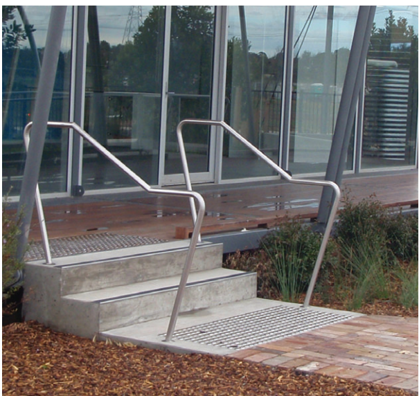
Compliant concrete stairs along pedestrian pathway with stainless steel handrails and tactile surface indicators compliant to AS1428.1.
