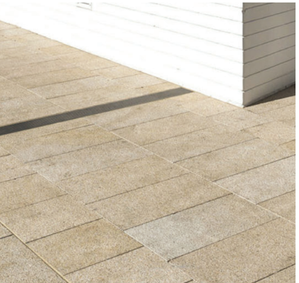
Primary surface treatment to be stone unit paving installed on mortar bedding and reinforced concrete base slab. Contrasting stone colour and texture will be used selectively throughout.
