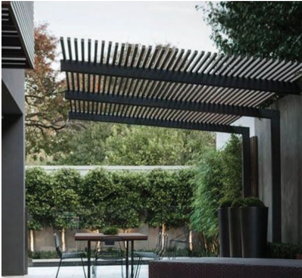
A cantilever shade structure will provide protection for the communal open space area. Steel frame with protective coating finish, hardwood timber battens.
